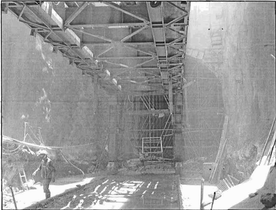
Erection of thlrđ skin of Gantry 2 through Surge shaft
