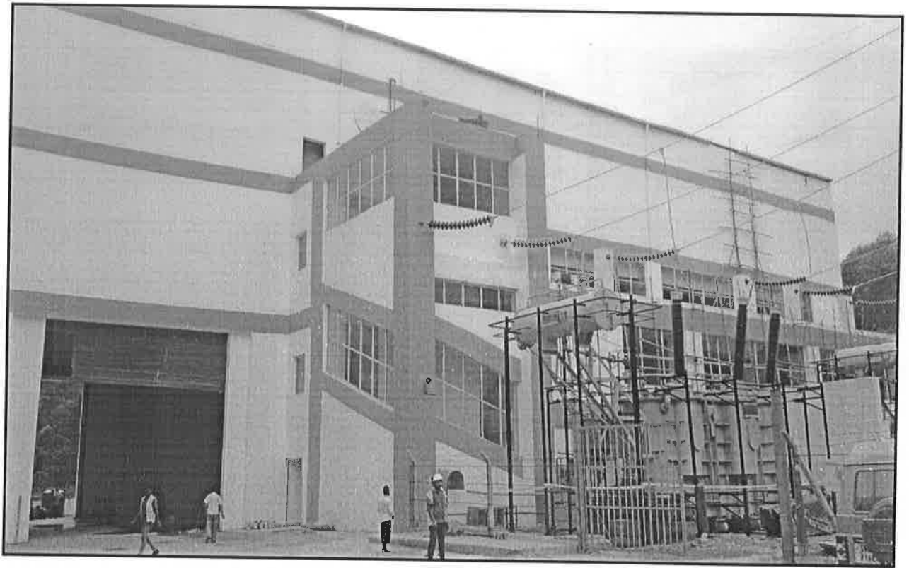
Power House U/S View
