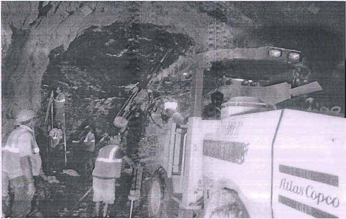
View of Face-3: Drilling work is under progress
