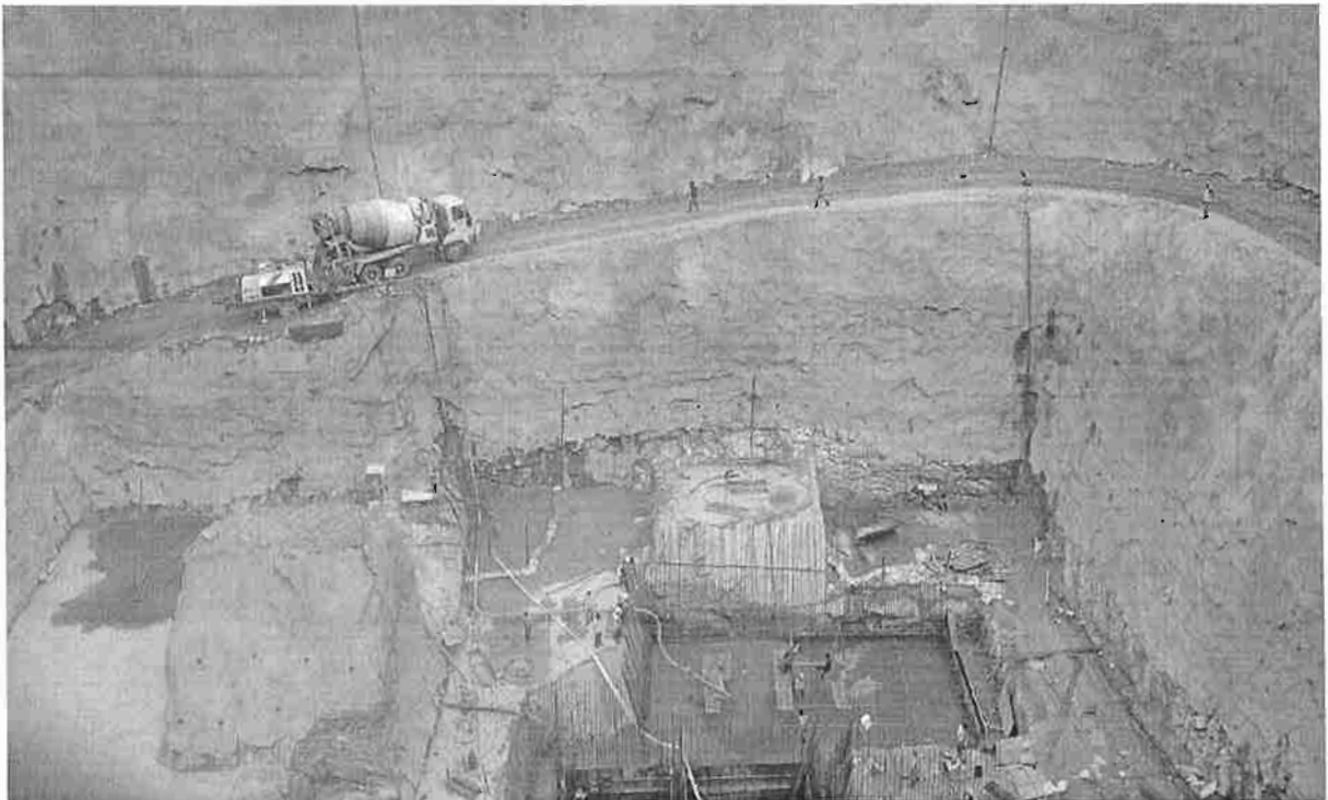
Concreting of Unit-2 raft under progress
