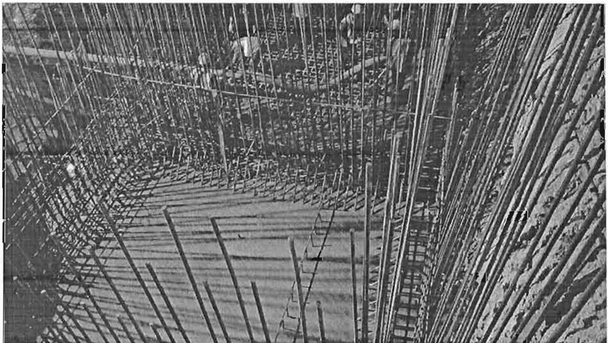
Concrete pouring in dewatering sum under progress
