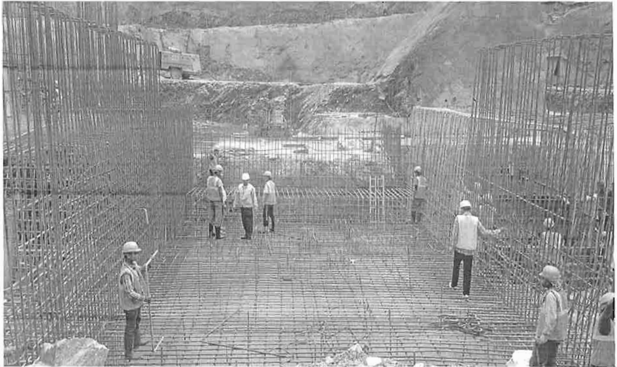
Reinforcement Binding of Unit-1 under progress
