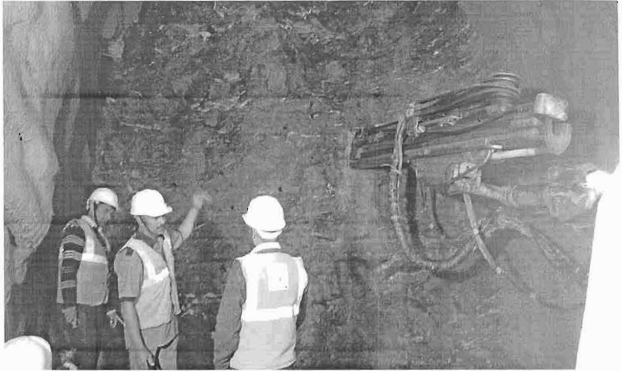
View of Face-5: Face drilling under progress
