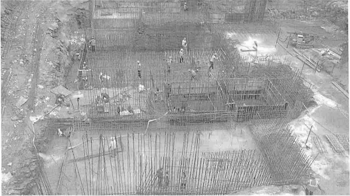
View of Power House reinforcement Binding
