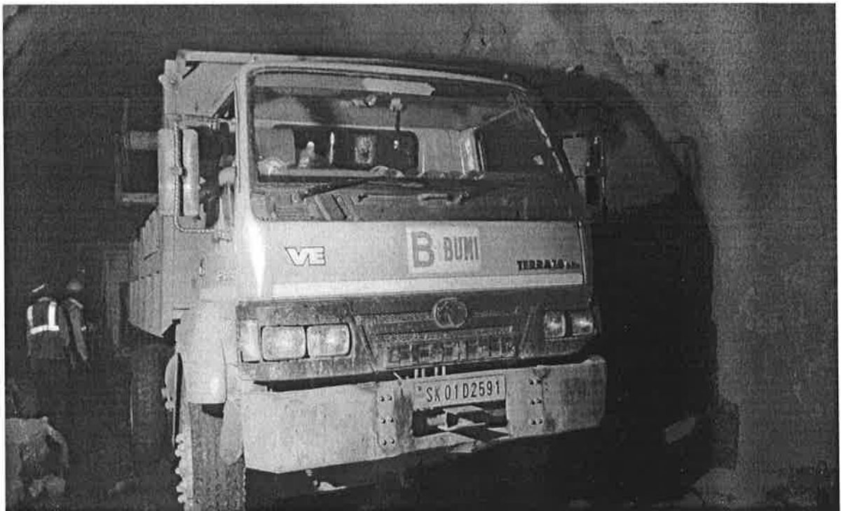
Penstock Tunnel-Mucking under progress
