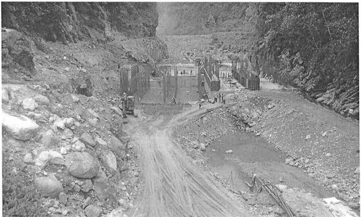
View of Barrage Works
