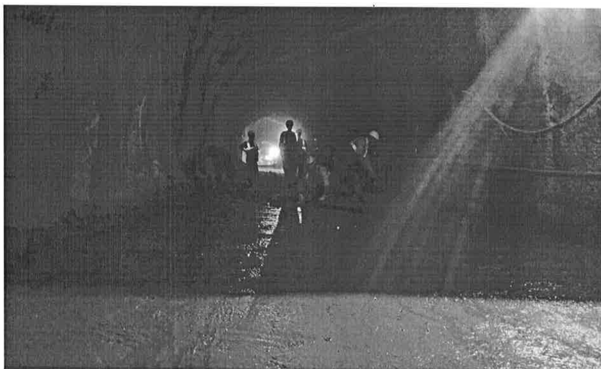
Pressure Tunnel Day-light
