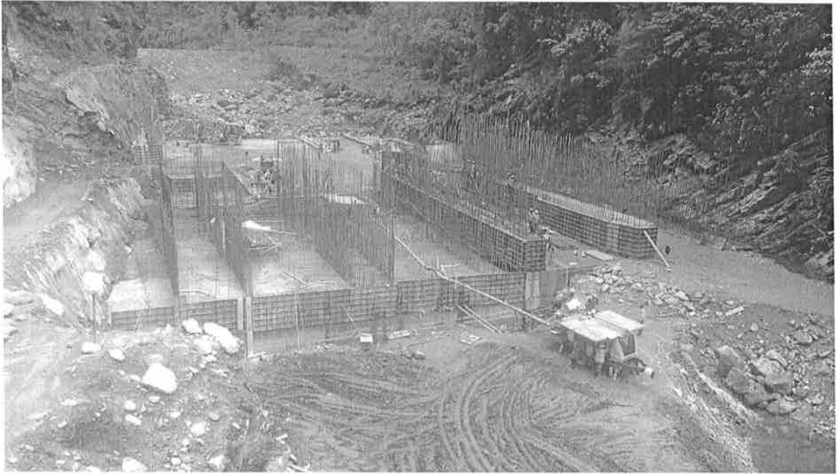
View of Barrage Works-Concreting of 2 nd lift under progress
